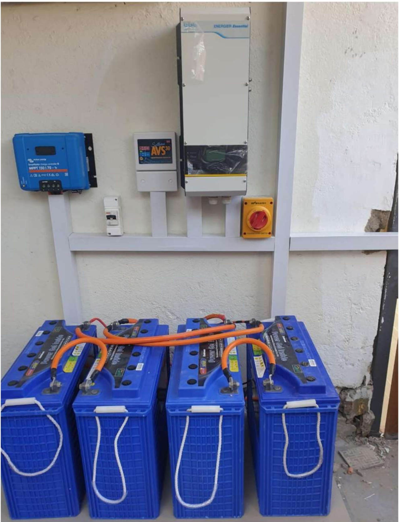
3kVA Inverter, 80A MPPT Charge Controller, 4 No. 200AH Deep-cycle Energy storage batteries & 2 no. 545W Solar PV modules system commissioned successfully in South C, Nairobi (September 2022)
