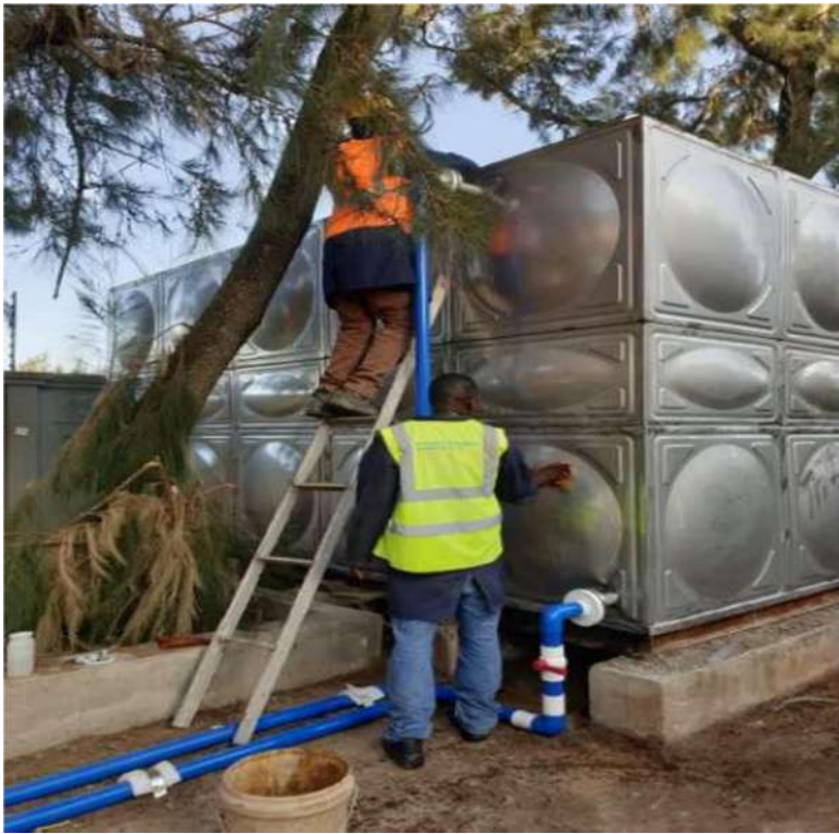
Structural & Construction works for a 50 cubic meters stainless steel water storage tank and the water filtration system installation works ongoing at the CRBC Office suites in Karen (January 2022)
