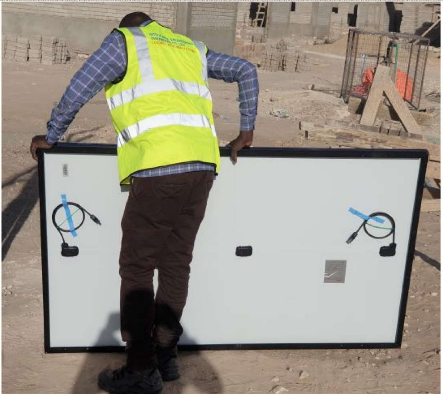
At Elwak, Mandera County. 20kWp Solar PV renewable Energy project ongoing, comprised of a 7.5kW Borehole Solarization & Water Pumping system and a 10kW off-grid Solar PV system for community water distribution.
