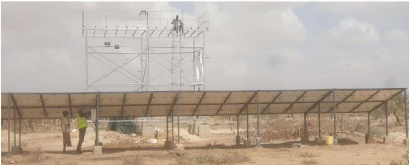
10 meters high elevated water tanks tower structural works ongoing alongside the electrical works for Solarization of 10hp Solar water pumping system in Habaswein, Wajir County, comprised of an 11kW Hybrid dual MPPT Inverter (March 2022)
